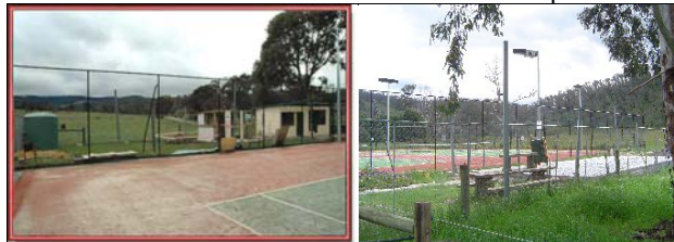
Demolition started in late September
