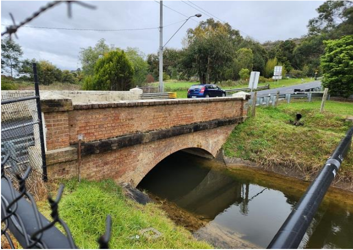
The red-brick arched heritage bridge over the Maroondah Aqueduct before recent road works (Photo from transport.vic.gov.au website)
