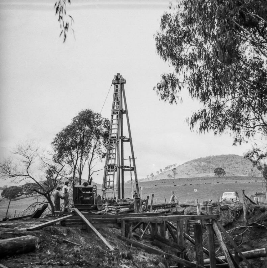
The old bridge looking eastwards. Pinnacle Lane, Steels Creek, Sep. 1955
